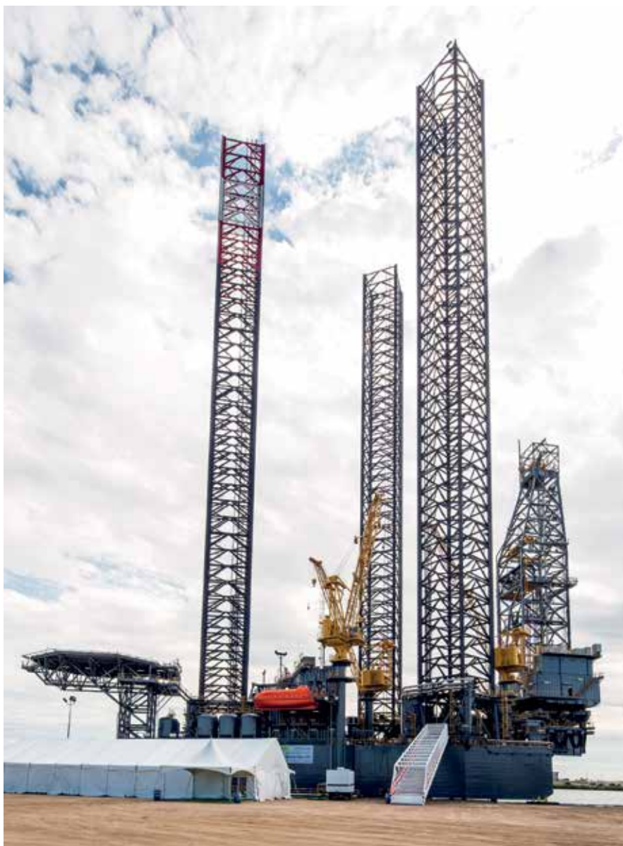
Keppel O&M has the expertise to build rigs of the LETOURNEAU™ design, having previously completed 16 such rigs, including the COATZACOALCOS, a LETOURNEAU™ Super 116E design which was built by Keppel AmFELS in Brownsville, USA
