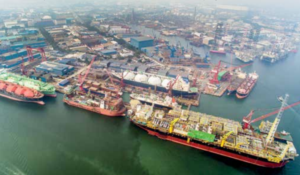
Work on the FPSO vessel, Cidade de Caraguatatuba MV27 (pictured in the foreground on the right at Keppel Shipyard, Tuas), leverages the synergy of Keppel's network of yards. After module integration work at Keppel Shipyard in Singapore, the vessel will depart for BrasFELS for further integration and commissioning works in 2Q 2016
